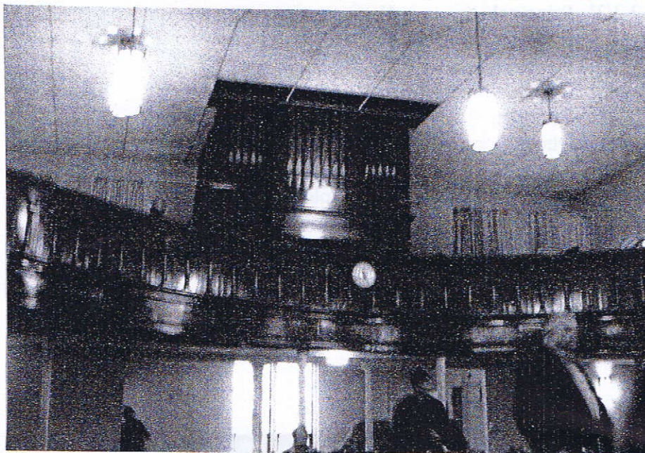
St. Paul's United Methodist. The organ stands in a traditional rear gallery. Ceiling has been lowered hiding the top portion of the instrument. Organ is in poor condition but it is all there. Photo: P. Birekner
